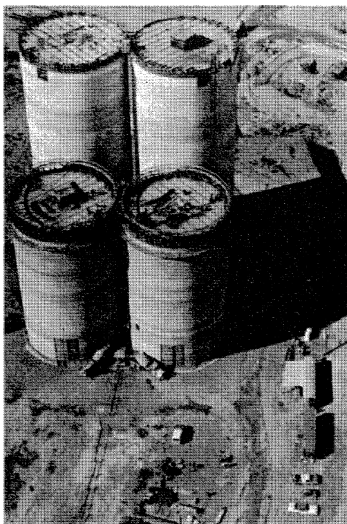
Figure 8.17. Aerial view—group of slip-form silos with silos in foreground under construction. (Permission First Colony Corp. and the Nicholson Co.)
